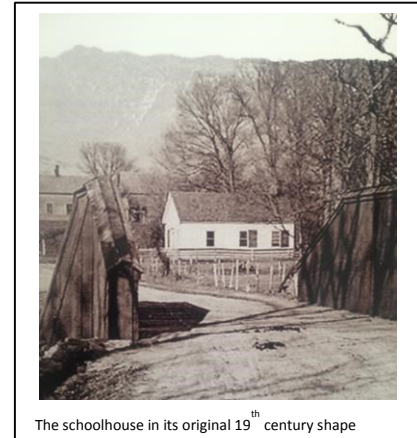
The schoolhouse in its original 19 th century shape
